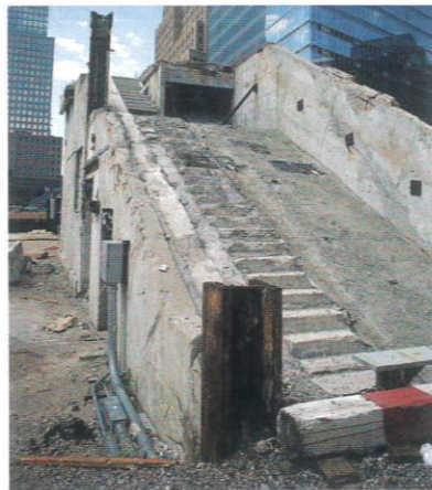
▲ Was it a miracle that 16 people survived in Stairwell B?
