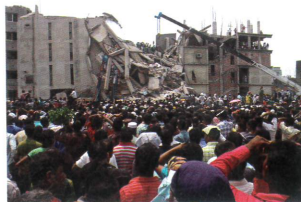
▲ The collapsed Rana Plaza factory
